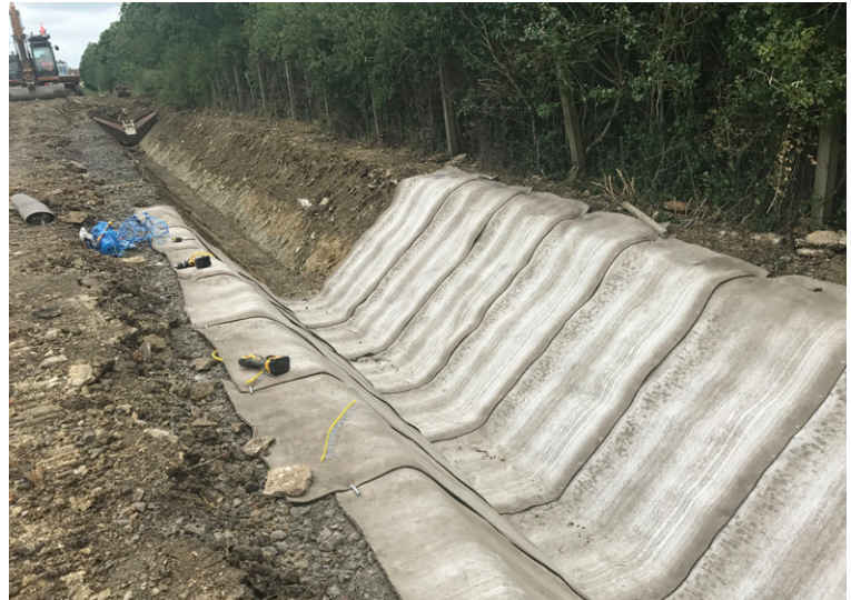
During installation, working upstream
