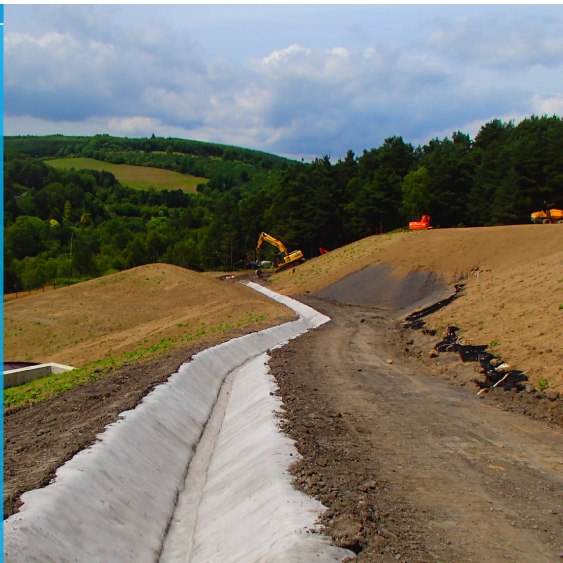
Overview of completed drainage channel
