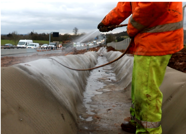
Hydration was given via hosepipe
