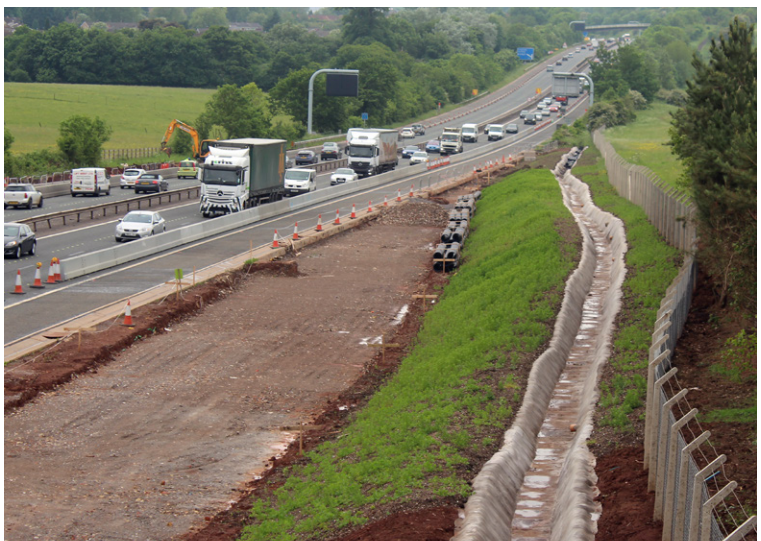
Completed installation and the surrounding area
