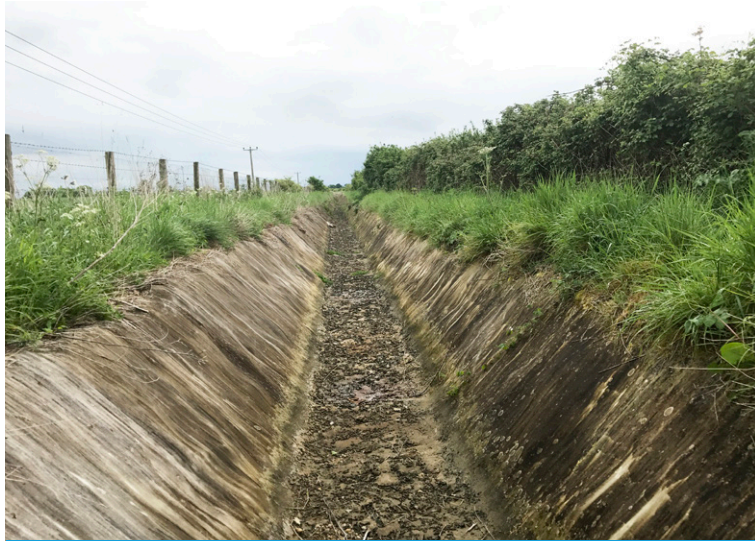
Original channel installed in 2014, 3 years after installation
