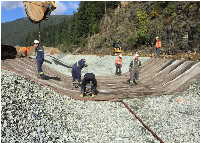
Screwing overlapped joints at 150mm centres
