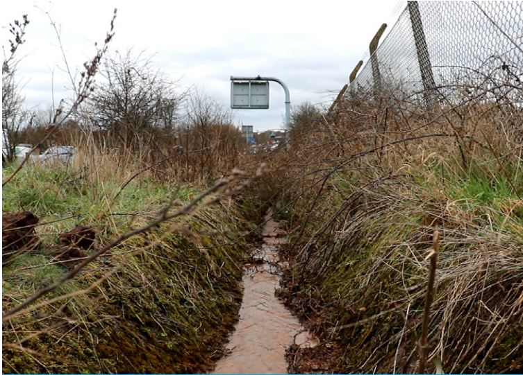
Channel before preparation
