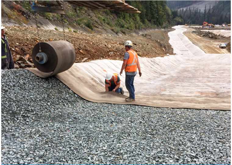
Dispensing of bulk roll CC8™ via spreader beam mounted onto excavator
