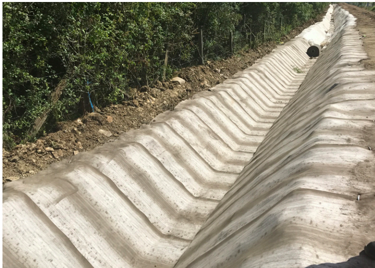
Installed CC prior to hydration and backfilling of anchor trench
