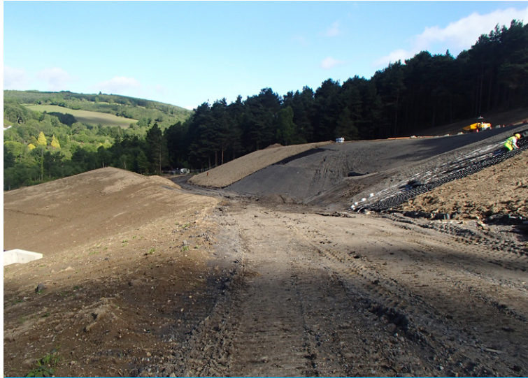
Site before installation of CC13™
