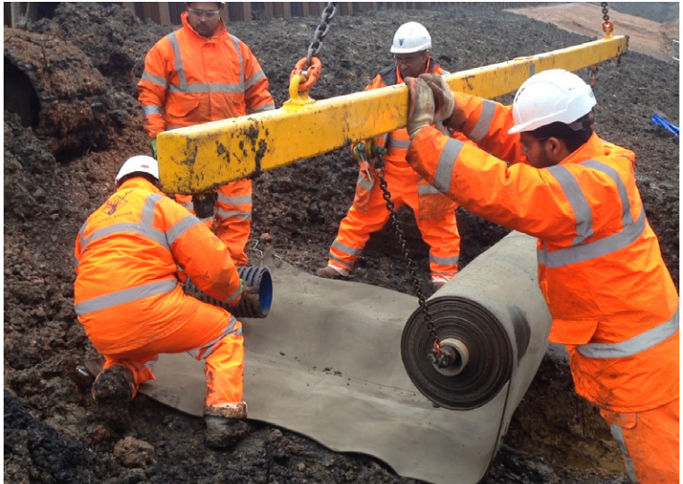
Steel pegs and screws were used to secure the CC
