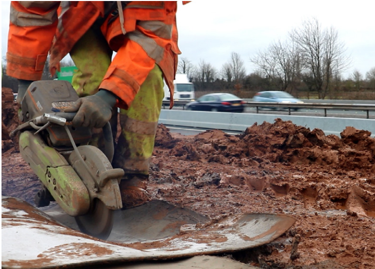
Hand power tools were used to cut the CC
