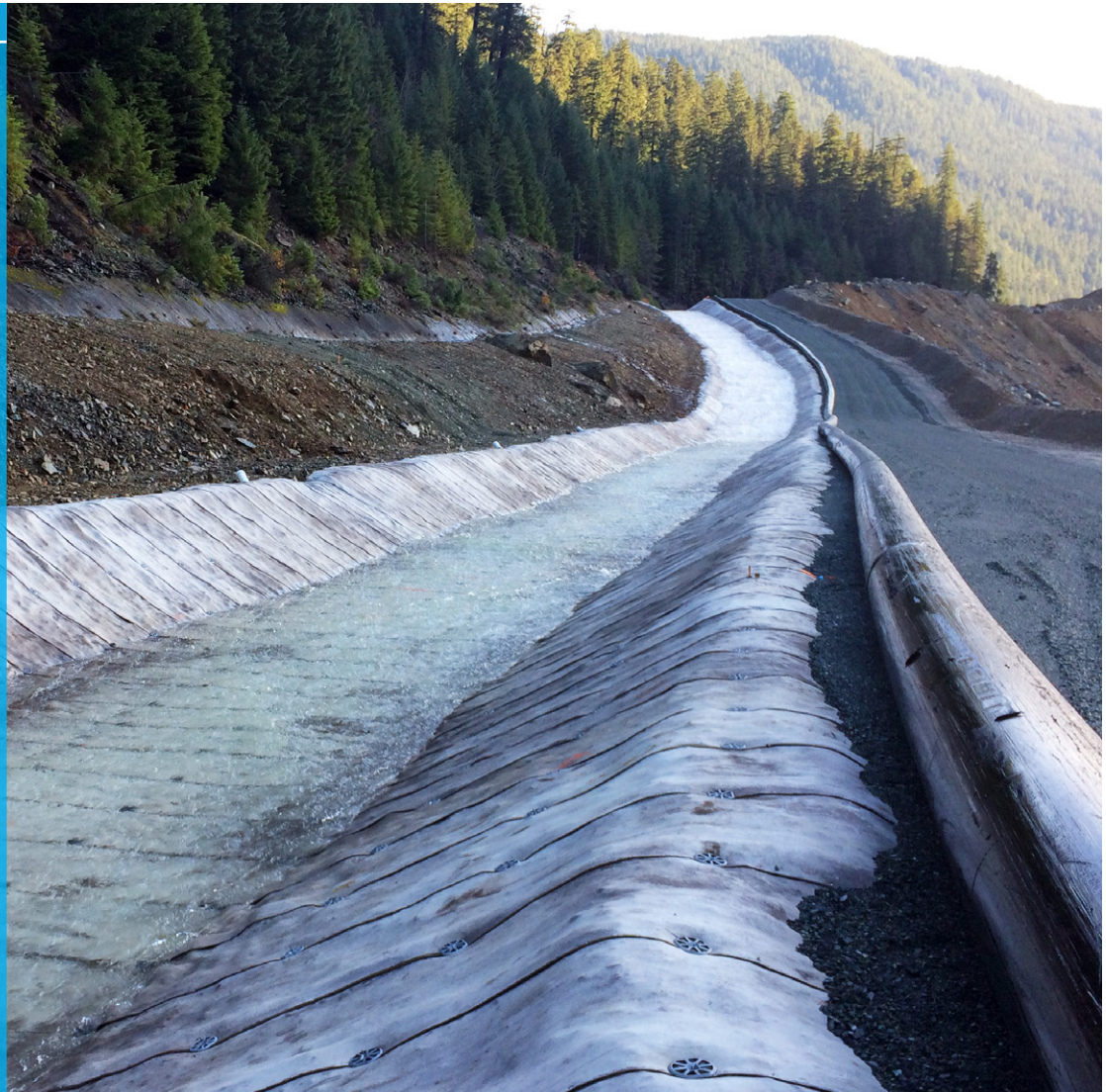
Completed CC lined channel with high flow 5 weeks after installation
