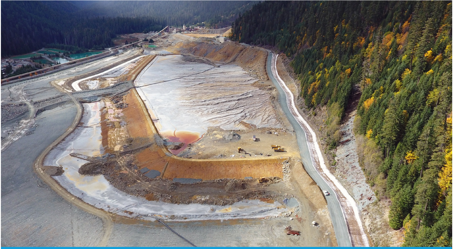
Aerial footage showing completed CC lined channel in relation to the mine
