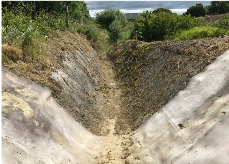
First layer of CC placed on existing concrete channel
