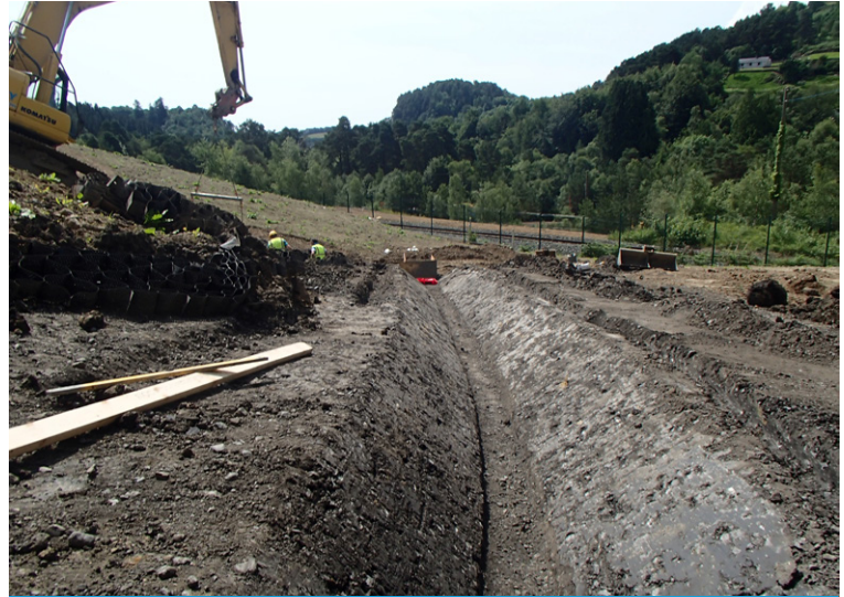
Channels prior to installation
