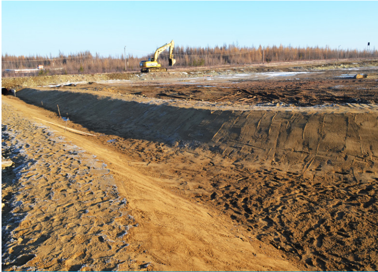
The excavated channel
