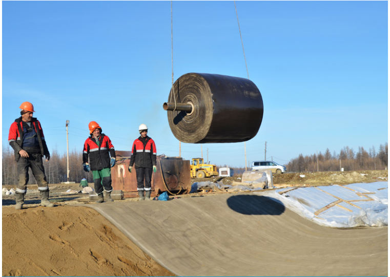
Bulk roll of CC13™ being lowered into position
