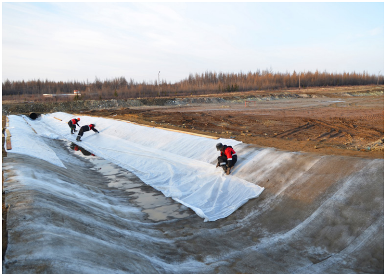
Protecting the CC with plastic sheeting
