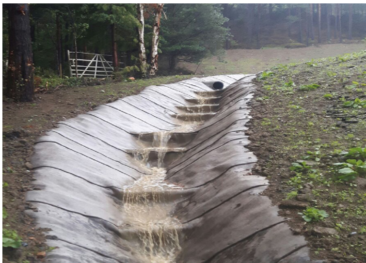
Completed installation in use
