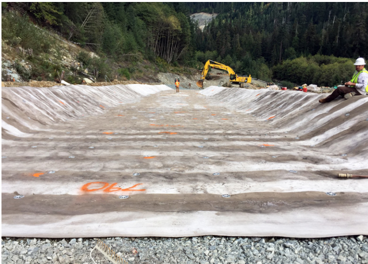
Spacing of percussion anchors through overlapped CC8™ layers
