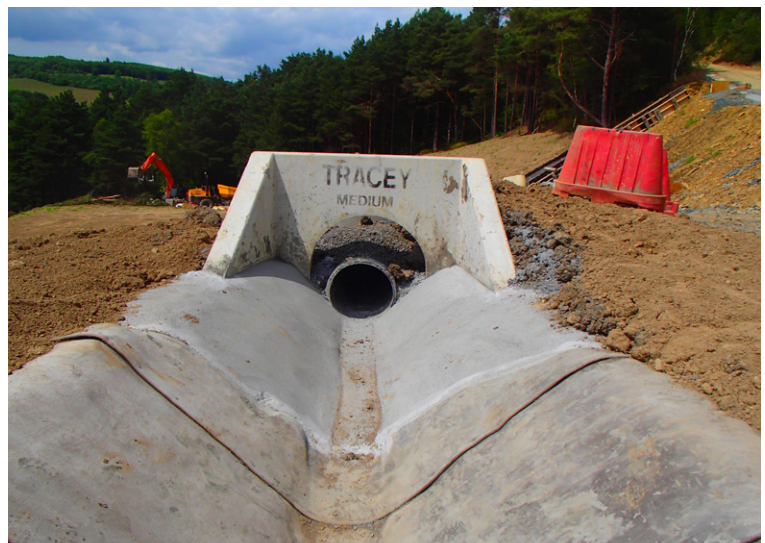
Headwall detail on upstream side
