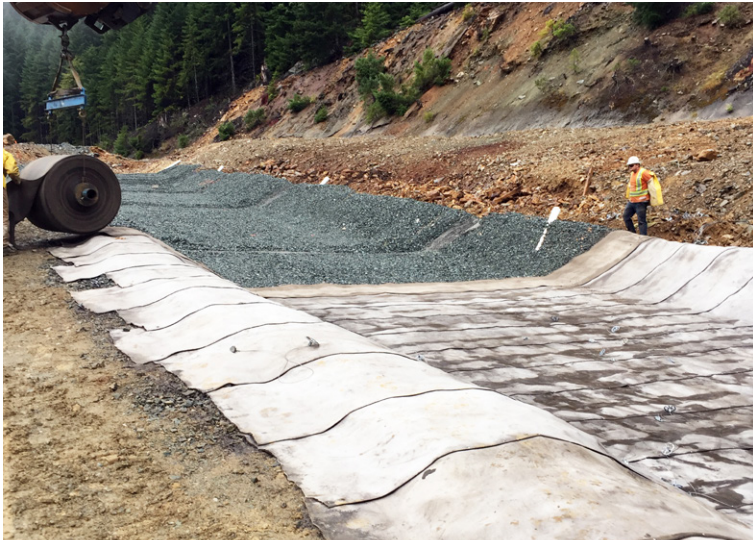
Anchor trench prior to backfilling
