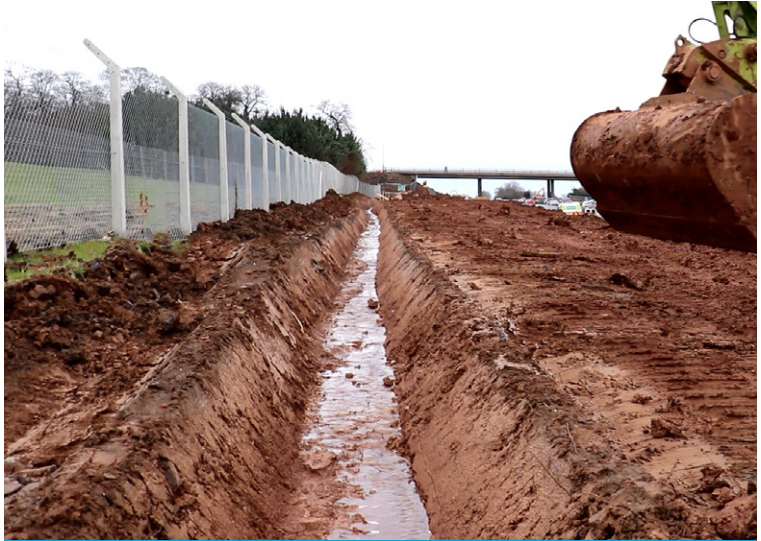
All vegetation and debris was removed before installation
