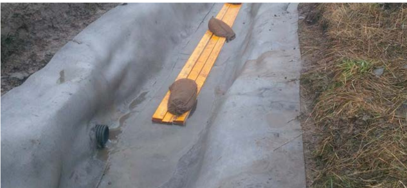
Weighing down the joints and a pipe penetration
