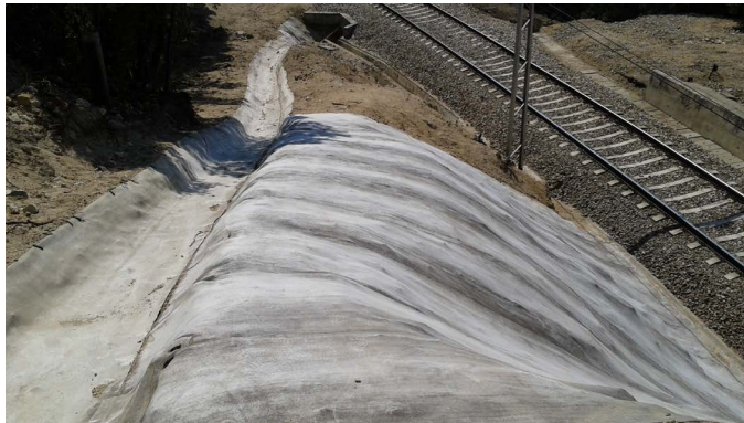
Ditch and slope interface
