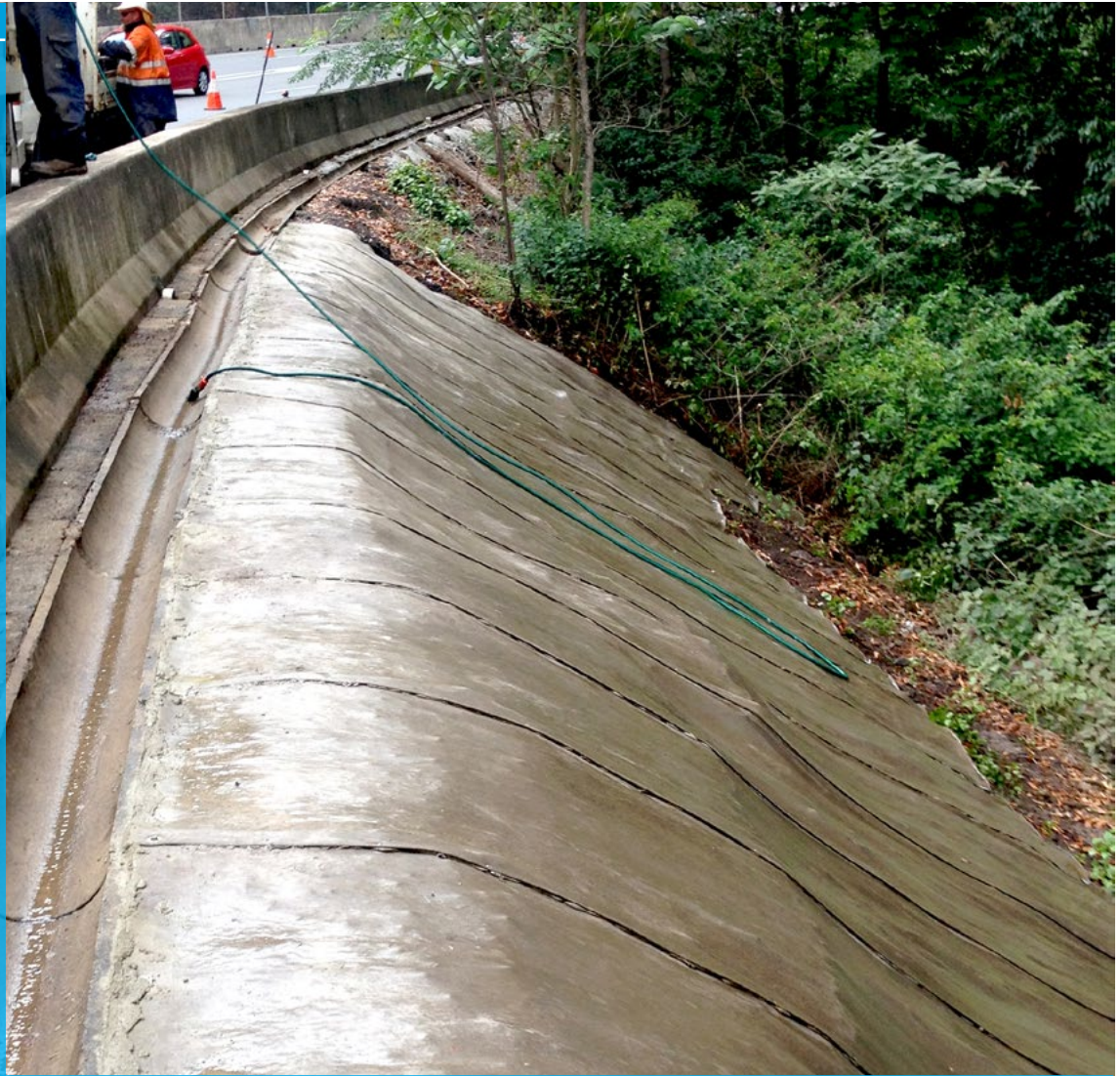
Section of slope immediately following hydration
