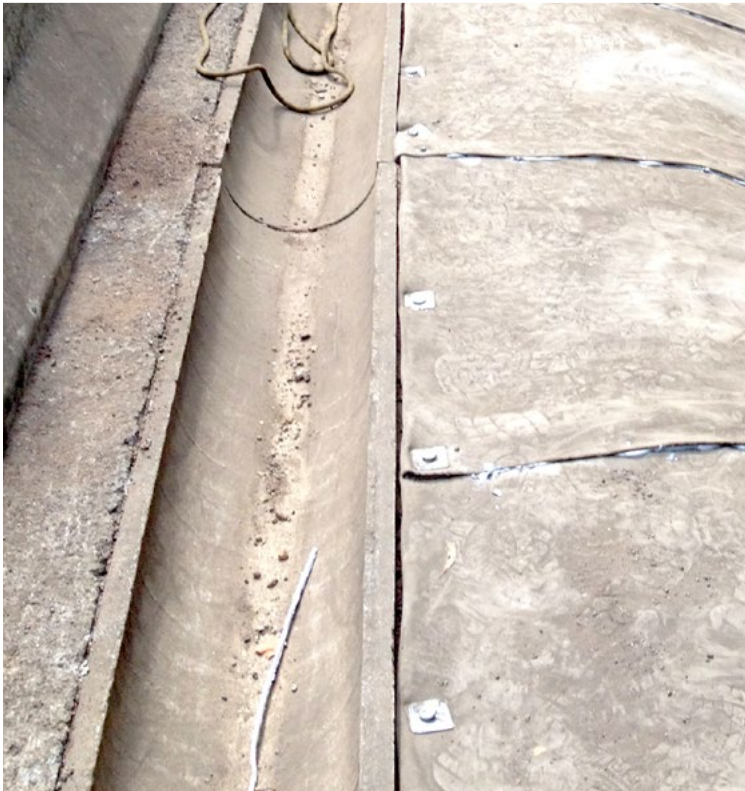
CC was fixed to the slope substrate using concrete anchors
