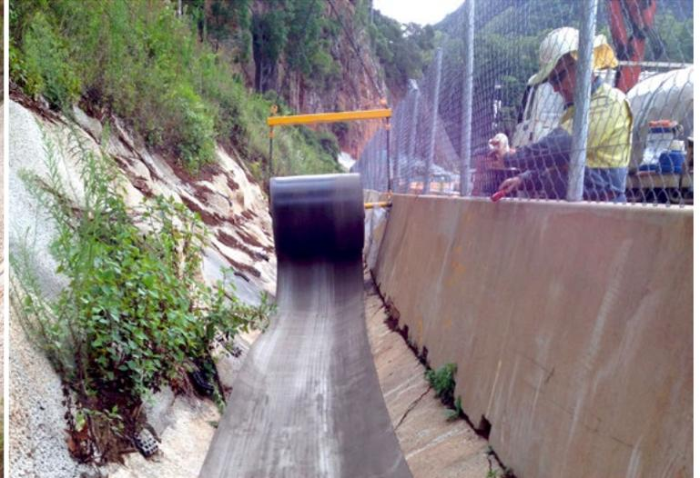
Bulk rolls of CC8 were dispensed using a spreader beam and crane truck
