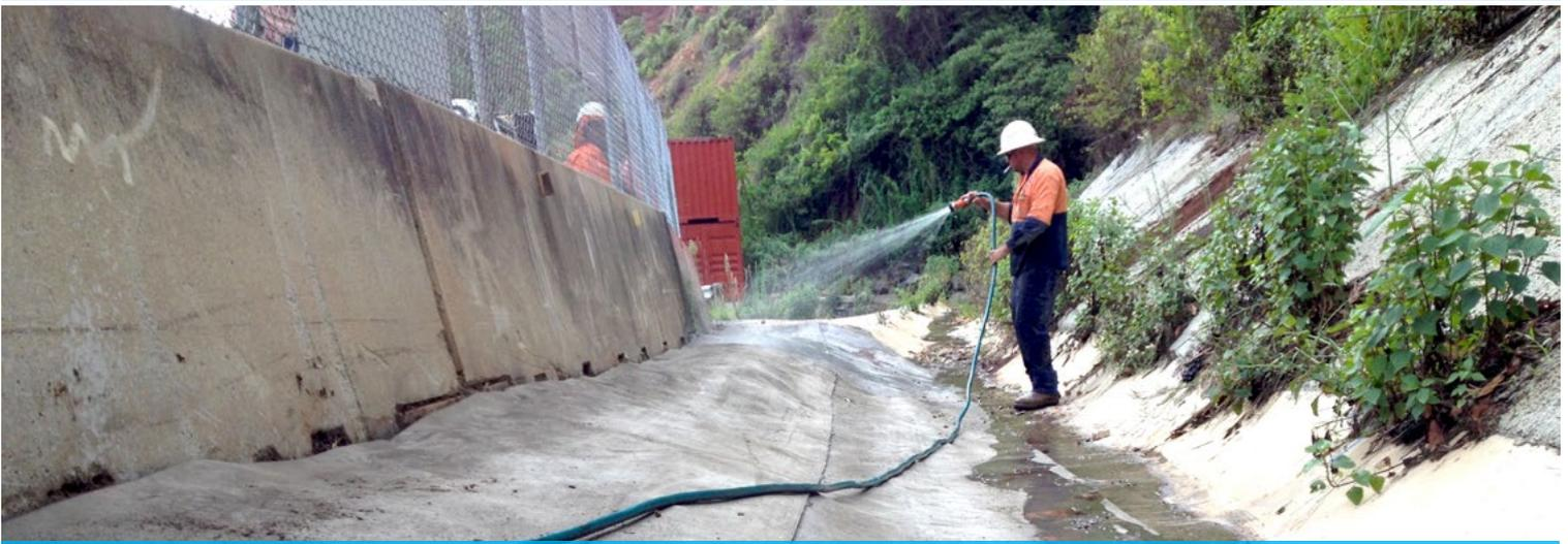
CC was hydrated using a water truck, pump and hose
