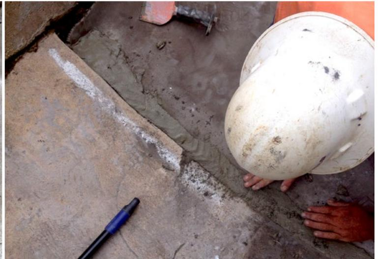
Grout was used at the end of the relined channel to prevent water ingress
