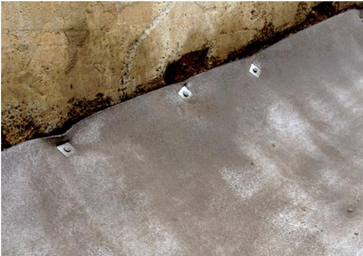
CC was fixed to the channel base using concrete anchors and screws
