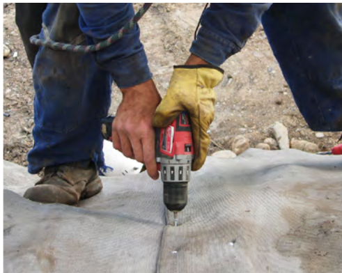
Joints were overlapped by 100mm and fixed with screws at approximately 200mm intervals.
