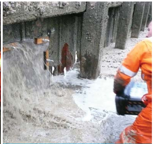
Hydrating the CC section with sea water
