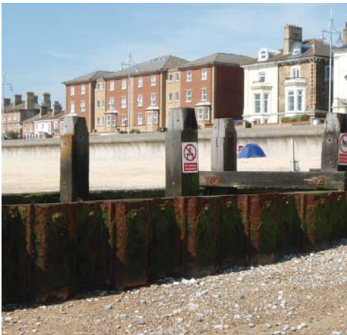
Steel pile beach groyne, Lowestoft
