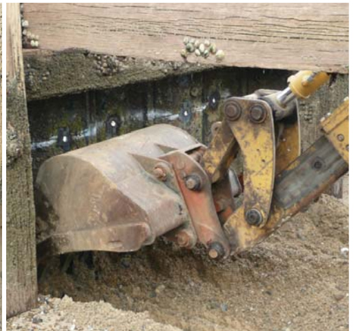
Excavating groyne section
