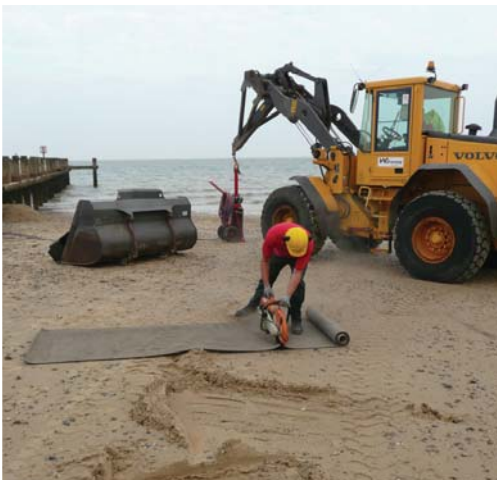
Cutting CC13 on site
