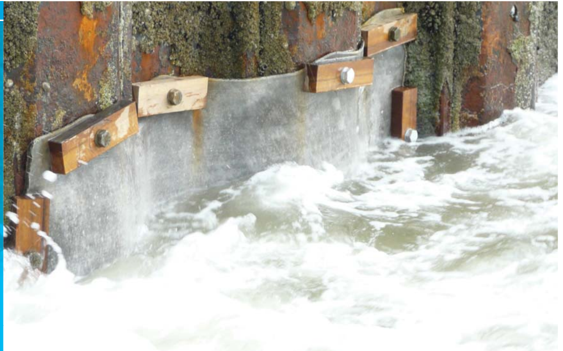
Completed repaired groyne section at high tide
