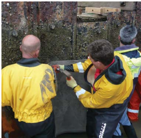
Bolting CC section to groyne
