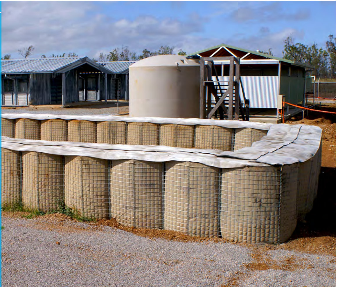
Completed gabion capping
