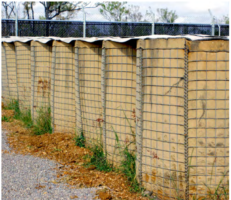
CC cap provides protection from inclement weather and high winds
