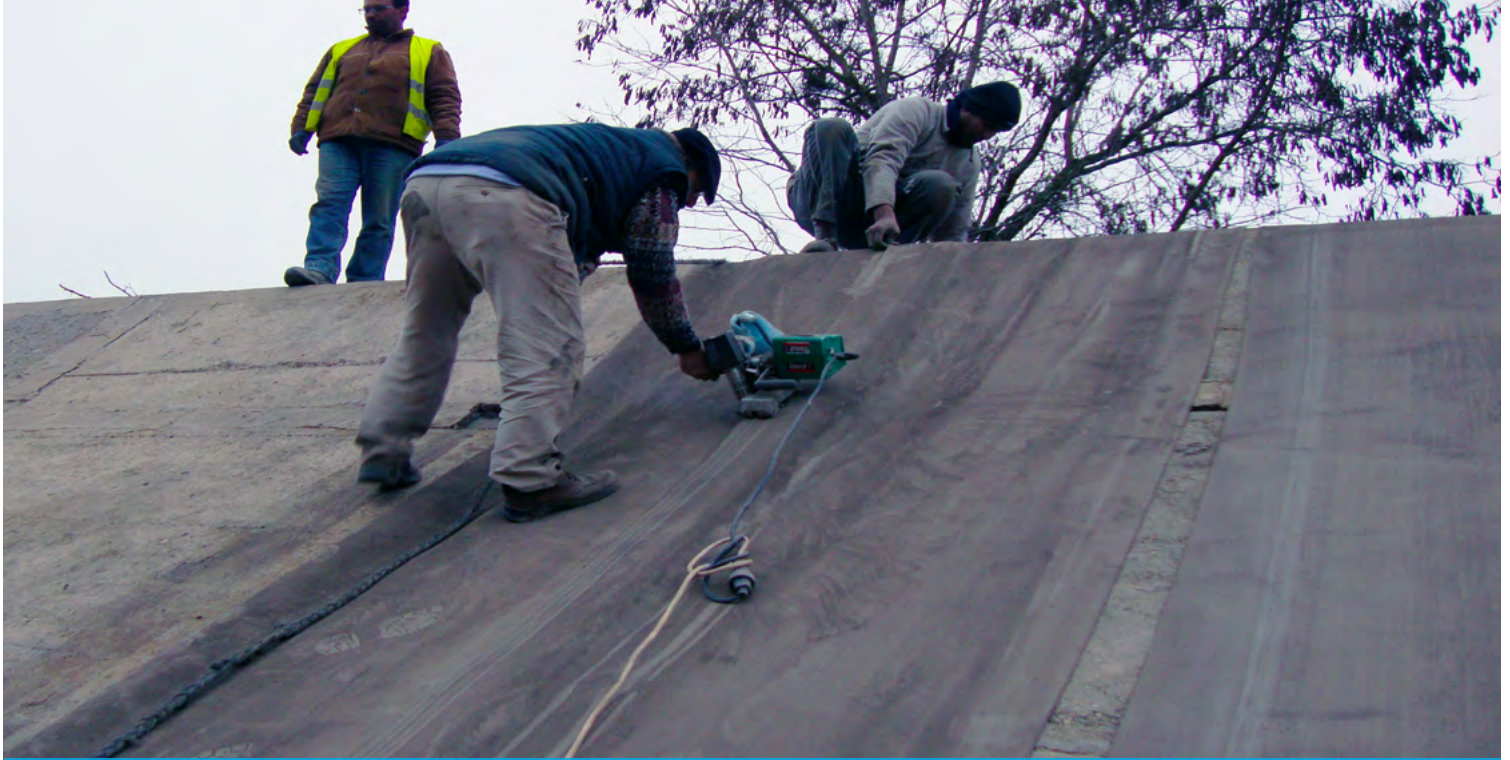
CC can be thermally welded, enabling it to provide waterproof protection.
