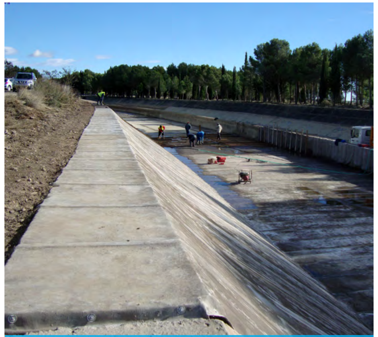
CC was secured at the crest with Hilti DBZ Wedge Anchors
