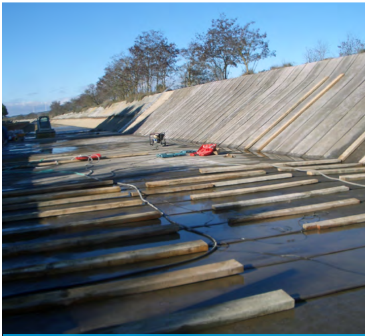
Thermally welded joints held flat during setting with wooden boards
