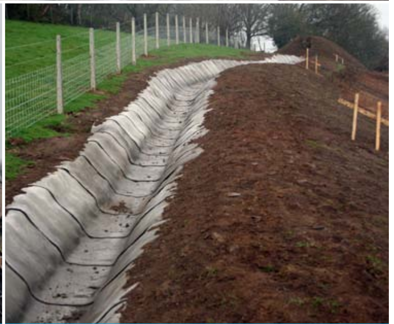
CC8 pre-cut layers laid transversely and in the direction of water flow.
