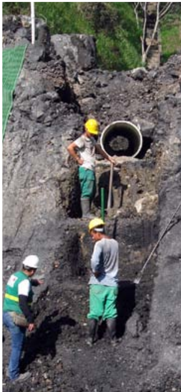
Grading and stepping of slope
