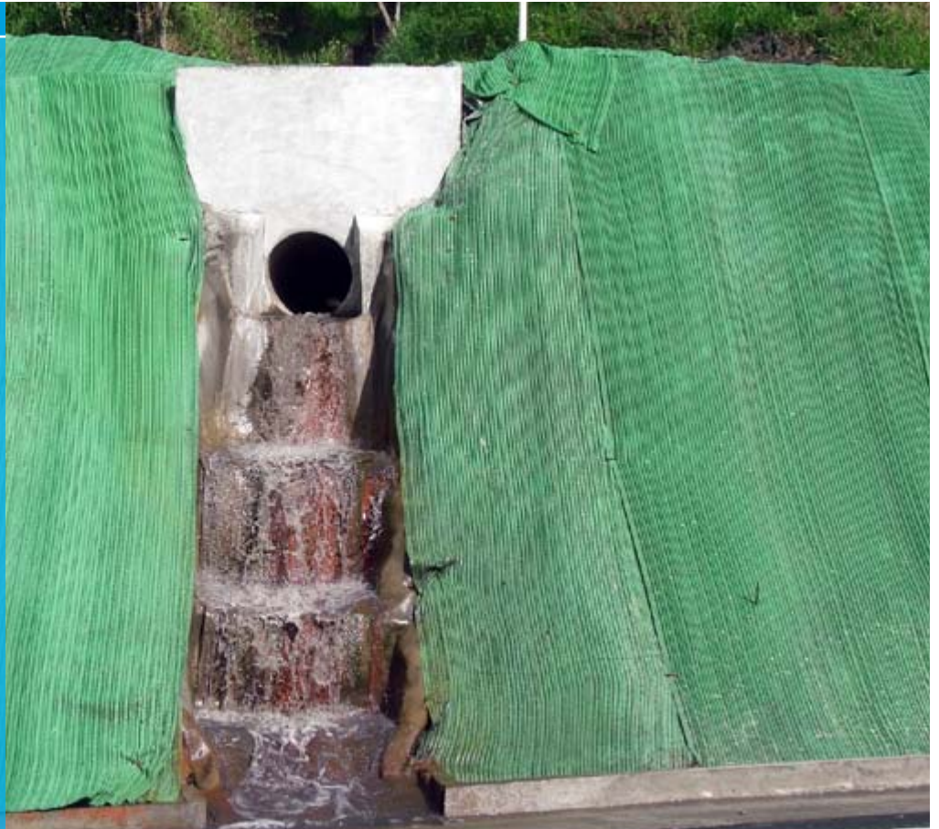
Completed CC lined dissipater drain
