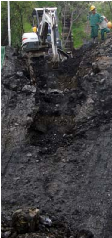
Excavation of slope
