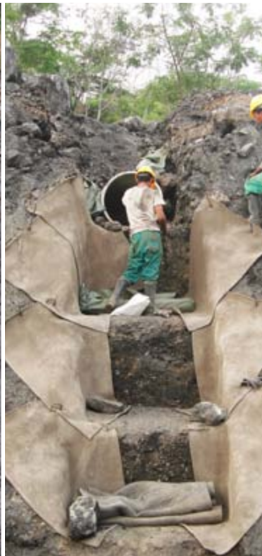
Fixing vertical CC sections
