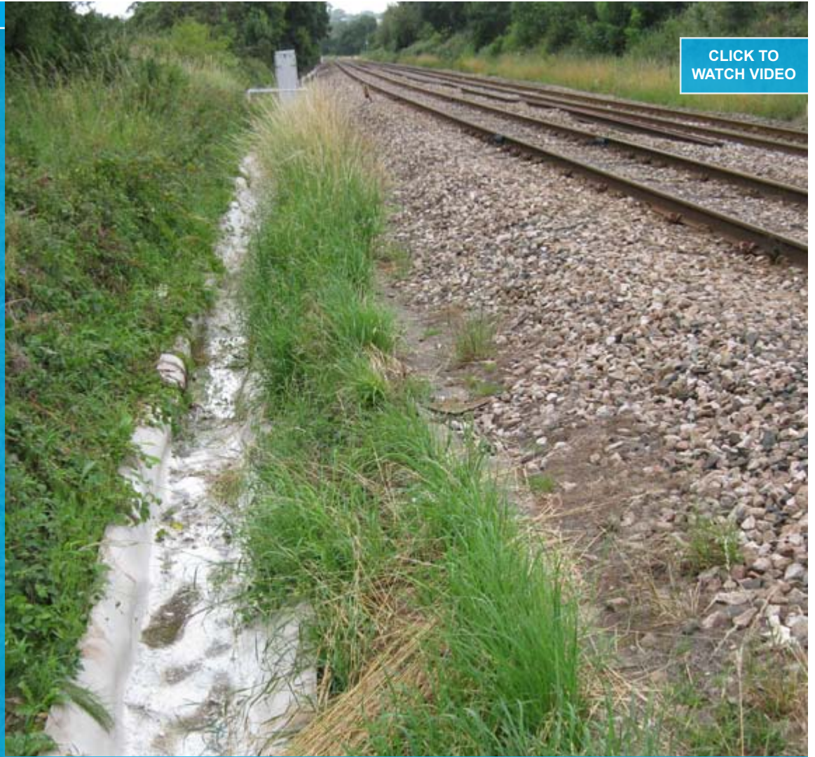
Completed lined carrier drain
